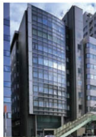
A-5 COI Higashi-Nihonbashi Building
