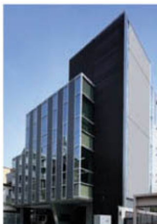
A-18 COI Shibuya Kamiyacho Building
